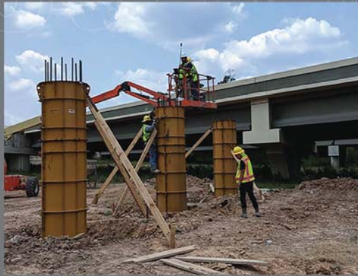
Construction - Segment H
