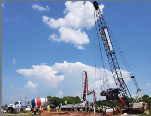
Construction - Segment I - 2B
